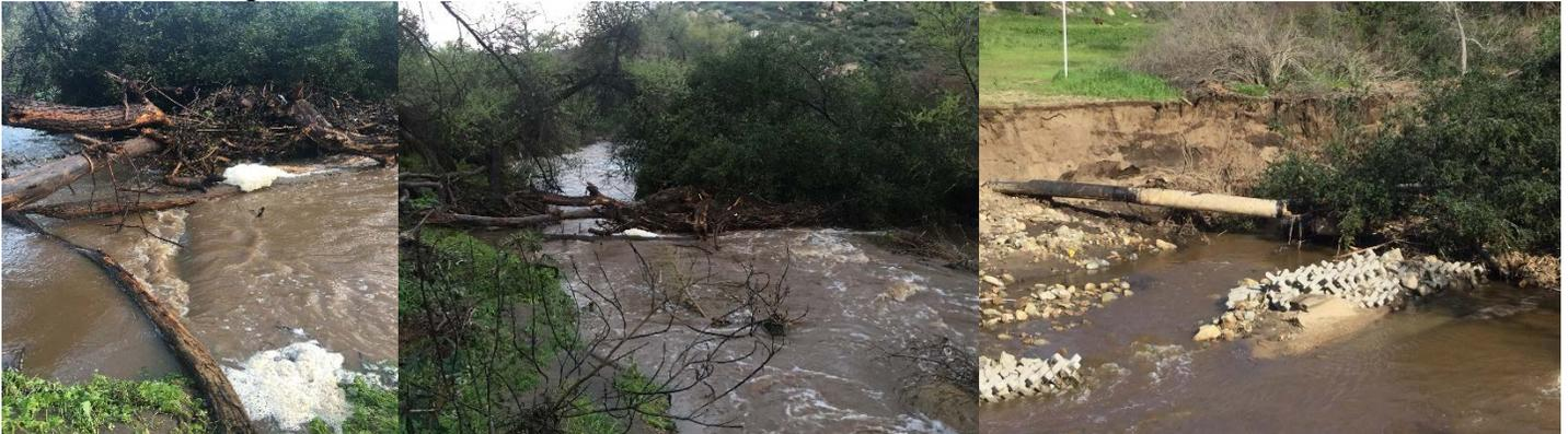
The District's supervisory control and data acquisition (SCADA) system registered an increase in flow of about 5000 gallons per minute just after 3:00 A.M. Fortunately, the increase was detected by an alert District staff member who happened to be making other adjustments to our system at that time (yes, this is truly a 24/7/365 operation). It was determined that the Moosa Crest Line was the cause of the spike and crews were able to isolate the pipeline rapidly, minimizing water loss.
