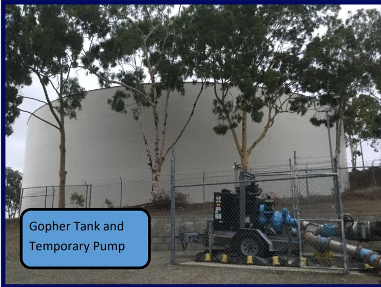
Morro Reservoir then feeds into three other storage facilities (Hutton, Gopher, and Turner tanks), with temporary pumping facilities. The tanks are monitored 24/7 and the levels are checked constantly to make adjustments throughout the day, forecast demands, and detect anomalies as they occur.
