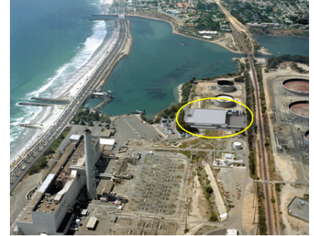
Poseidon Water Treatment Site-Carlsbad
