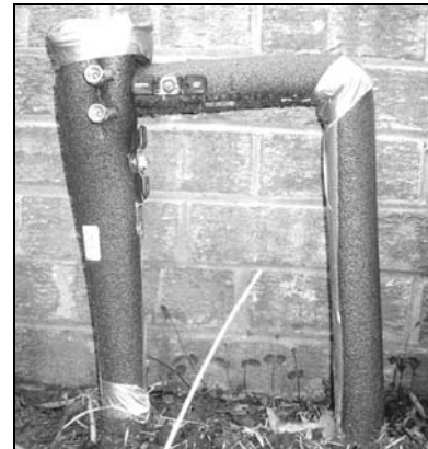
Insulated Backflow Device
