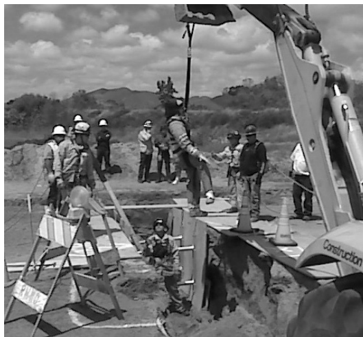
Crews Lifting Training Dummy
