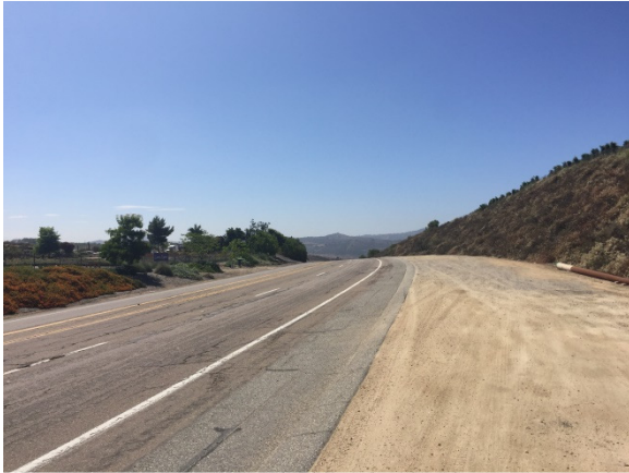
Looking southeasterly along Old Highway 395; Subject to right
