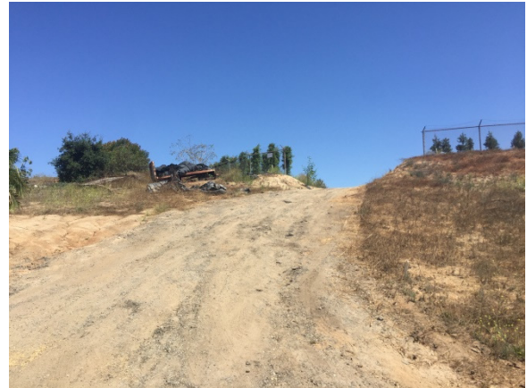
Access into reservoir
